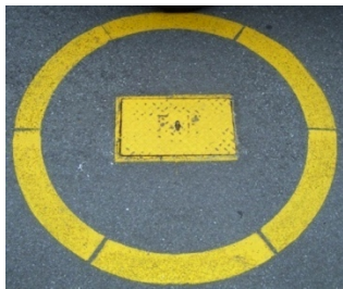
16-7 - Fire Hydrant marking
