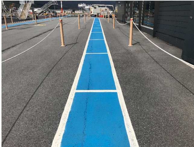
16-10 - Passenger Walkway line
